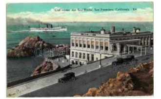
21712. * San Francisco, Cliff House, Seal Rock T31000
