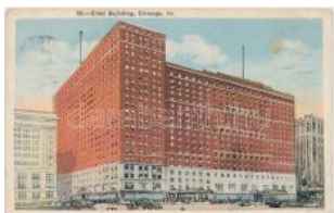
21634. ☒ Chicago, Eitel Building (EK) T2/3 1000
