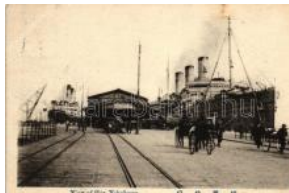
22199. ✱ Yokohama, Pier T2 1600
