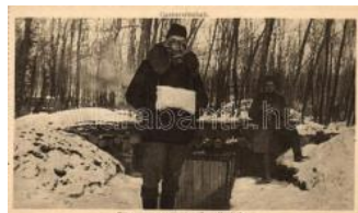
23419. ✱✱ 1944 WWI Prep aration for the occu T2/31400
