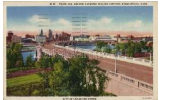
21666. ☒ Minneapolis, Third Ave. Bridge, Showin T21000
