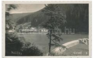
21365. * Martalja, Vízmu / water plant T2 1200
