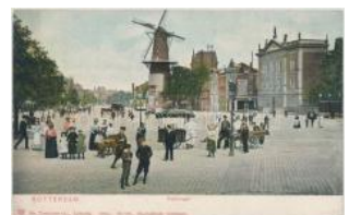
22140. ** Rotterdam, Coolingsingel square, mill T1/2 1400
