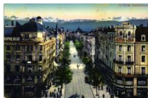
22907. ** Zürich, Bahnhofstrasse / railway station T2 1400
