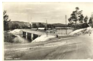
22918. * Sorsele, Lillabron / bridge T2 1000
