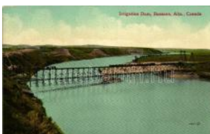
22205. ✱✱ Bassano, Irrigation dam T2 1200
