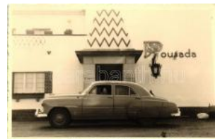
22844. * Elvas, Hotel Pous ada, photo T2 1000
