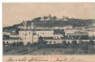
22590. ☒ Conegliano, railw- ay station (cut) T4 1400
