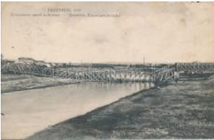
22257. ☒ Przemysl destroyed railway bridge (b) T4 1400
