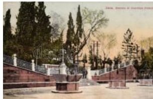
21550. * * Zadar, Zara; entry of the Public Gallery T2/31400
