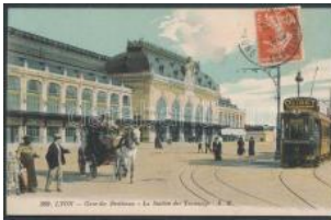
22100. ☒ Lyon Brotteaux railway station, tram T1/2 3000
