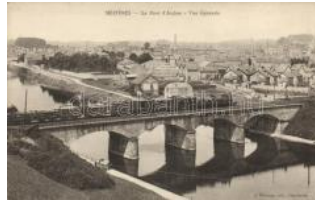
22110. ✱✱ Mezieres (Charleville) railway bridge T1/2 1400
