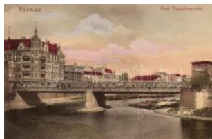
22213. ** Poznan, Most Chwaliszewski / bridge T2/31600
