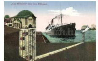
22360. ✳✳ Hamburg, Elbtunnel, SS Cap Finister T21000
