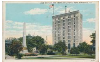
21817. ☒ Pensacola, Plaza and American National Hotel T2/3 1000
