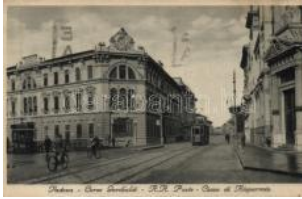
22497. ☒ Padova, Garibaldi's street, post office, T2/31400
