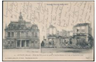
22138. * Revigny Town Hall, before and after b T2/3400
