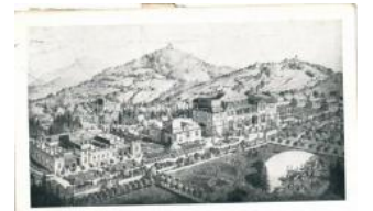
21751. ☒ Versec, Vrsac, Sanatorium sanatorium T2/3 1400
