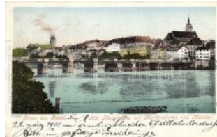
22619. ☒ Basel bridge, Mar tin church (EK) T2/3 1000
