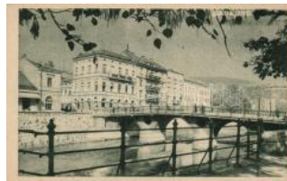
22607. ✱✱ Sarajevo, bridge T1/2 800
