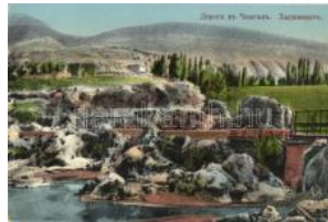
23355. ✳✳ Hodzhikent, Road to Chimgan T2 1000
