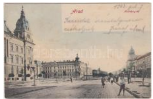
21671. * Arad, Andrássy tér / square (wet damag) T4 600
