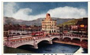
22734. ** Kyoto, Shijoohashi, bridge, tram (E T2/31200)
