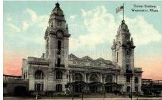
22522. * Worcester, Union Station (EK) T2/3 1000
