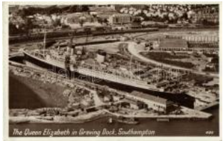
22913. ☒ Southampton, Graving Dock, RMS Que T21000
