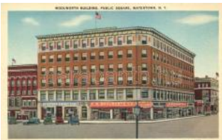
22197. ** Watertown, W oolworth Building, Pu T11000
