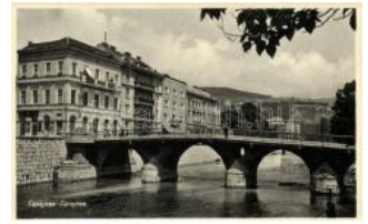
22304. * Sarajevo, bridge T1/2 1800
