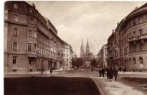
21883. ** Zagreb, Ulica Rackoga / street (fa) T3/41200
