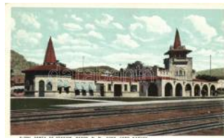
22143. ✱✱ Raton, New Mexico, Santa Fe Station T2/3 1600
