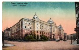
22319. ** Brno, Brünn; jus tice palace T2 1200
