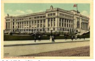
22173. * St. Louis, Missouri; Municipal Building T21200
