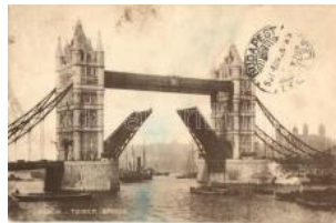
22679. * London, Tower bridge, ships (EK) T2/3 1000
