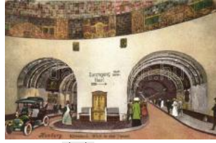
22755. ✱✱ Hamburg, Elbtunnel / Elbe Tunnel T2 1600
