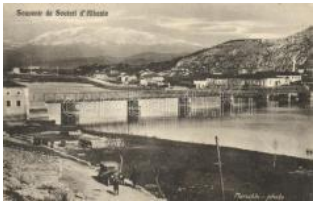
21977. ** Shkoder, Shkodra; Scutari; bridge, T1/22600
