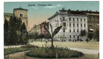
21909. ✱✱ Zagreb, Trenkova ulica / street T2 1400
