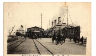
22462. * Yokohama, Pier T2 1600
