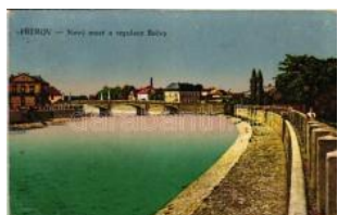
22264. ☒ Prerov, Bečva river, bridge (EK) T2/3 2600
