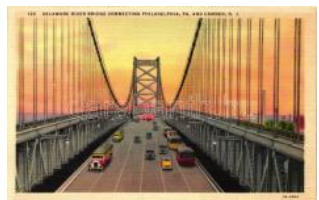
22007. ** Delaware river bridge connecting Ph T1 1600
