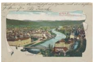
22107. ☒ Graz, Ferdinandsbrücke / bridge T2/3 1000
