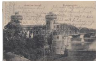
22716. 1891 Mainz, Eisenbahnbrücke / Railway bridge T2 1400
