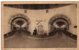
22687. ** Hamburg, Elbtunnel / Elbe Tunnel (E T3/4) 400
