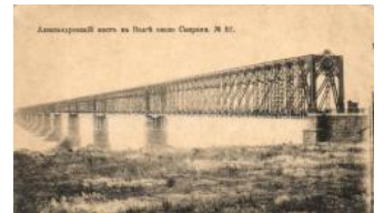
22914. ** Syzran, Alexan der Railway Bridge o T3 1000
