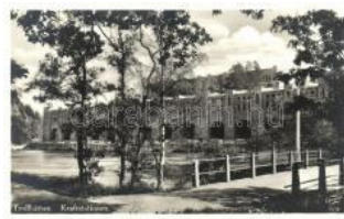
23184. * Trollhattan, Kraftstationen / power station T1/21000
