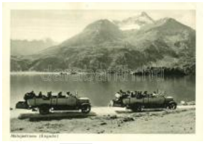
23135. ** Engadin, Malojastrasse / road, sign T2/3/2000
