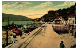
22800. ☒ Herceg Novi, Cas telnuovo; railroad, po T32200
