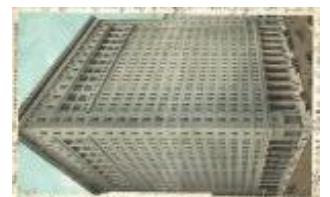
22434. ✱ Chicago, Peoples Gas Building, autom T3 1000
