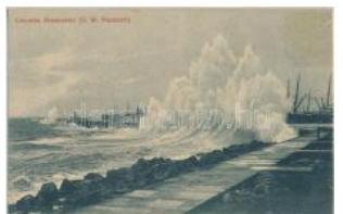
23117. * Colombo Breakwater (S.W. Mousson) T2 1200
