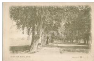
22477. * Perth, South Ingham Avenue T2/3 1000
