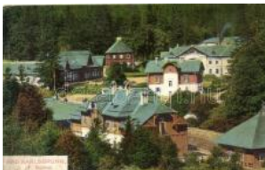
22599. ** Karlova Studánka, Bad Karlsbrunn T2/31000
