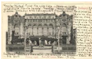
20565. ☒ Budapest V. Viga-dó T1/2 800
