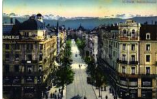
23164. ** Zürich, Bahnhofstrasse / railway station T2 1400
