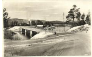
23177. * Sorsele, Lillabron / bridge T2 1000
