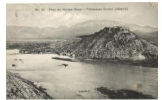
22418. ✱ Shkoder, Shkodra; Fortress (Rb) T3/4 1000
