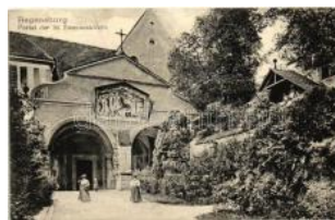
22949. ☒ Regensburg, Portal of St. Emmeram's Church T21400
