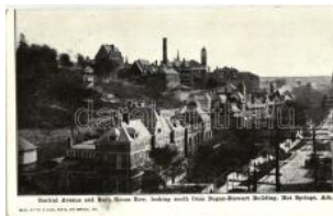
21313. ** Hot Springs, Arkansas; Central Avenue T2 1200
