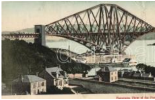
22015. * Forth Rail Bridge panoramic card (bent T3) 2000
