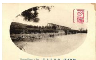
21844. ** Ise, Railway bridge T2 1200
