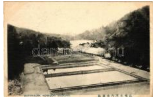
21856. * Nagasaki, Honkoc hi, water work T2 1200
