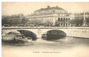
21717. ** Paris, Theatre d u Chatelet, bridge, T2/3) 1000
