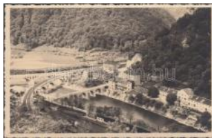
22473. * Zidani Most, bridge T1/2 1400
