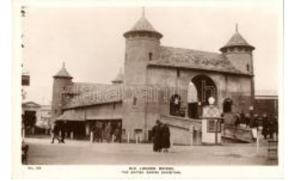
23094. ** London, Old bridge T1 1000
