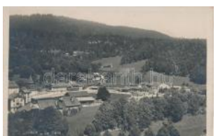
23352. ** Saint-Cergue, Gare / railway station T2 1200
