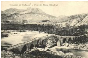
22541. * Shkoder, Shkoder; Pont de Messi / bridge (EK) 2000
