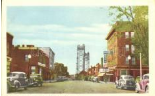
22987. * Welland, East Main Street and Lift Bridge 1200
