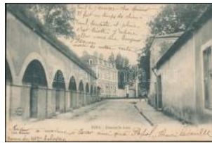
22953. ☒ Toul, Caserne St. Léon / barracks T2 1200
