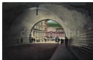
23257. ☒ Trieste, Montuza tunnel interior T2 1600
