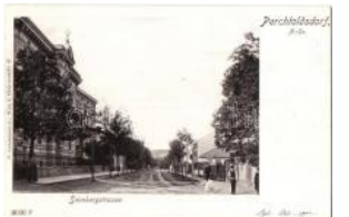
22679. * Perchtoldsdorf, Sonnbergstrasse T2 3000
