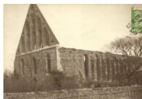
22916. * Tapa, destroyed church So. Stpl photo (E) 1400
