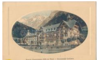
23168. ** Colle Isarco, Gossensass; Grosshotel G 1400
