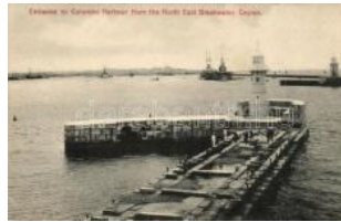
23293. ** Colombo, entrance to the harbour from 1200
