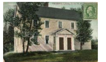
22562. * Dover, Old Quaker Church (EK) T2/3 1600
