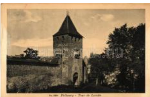
23323. ** Fribourg, Tour d e Lorette / tower T1/2 1600
