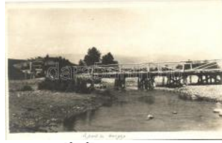
23280. ** Gorgop, bridge photo T1/2 1000
