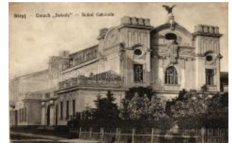
22137. Stryi, Stryj; Gmach Sokol / Sokol building 1600
