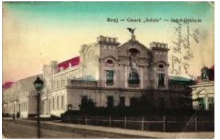
22138. Stryi, Stryj; Gmach Sokola / Sokol building 1600
