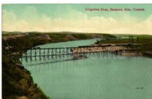
21570. ** Bassano, Irrigation dam T2 1200
