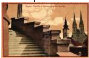
22009. ✱✱ Zagreb, stairs , Strossmayer promena 1200
