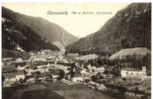
22153. ☒ Gusswerk, Eisengusswerk / view with iron 3000
