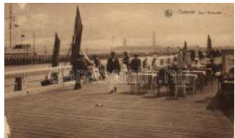
22258. * Ostend, Estacade / pier, boat (EK) T2/3 1000
