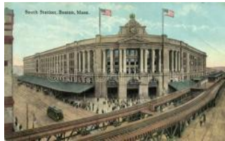
22078. ** Boston, Massachusetts; South Station ( 1400
