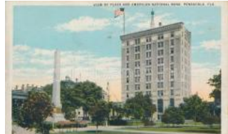
22110. ☒ Pensacola, Plaza and American National Bank 1000
