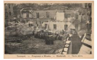
22850. * Ternopil, Tarnopol; Market place, damag 2200
