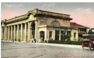
22667. ✱✱ Panama City, railroad station, automob 2000
