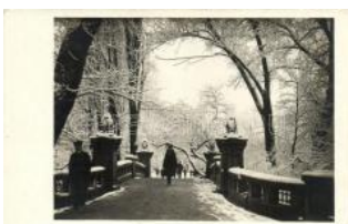
22707. * Bucharest, Cismig iu Gardens, bridge at w 1000
