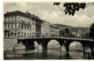
21933. * Sarajevo, bridge T1/2 1800
