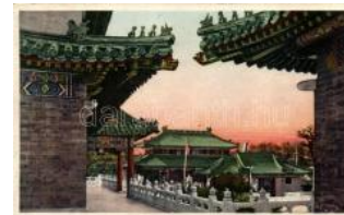
22190. * Beijing, Peking; College gatehouse and a building 1000
