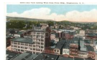
21830. * Binghamton, view from Press Building ( 1000
