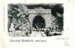
21571. ☒ Ruttkárol, Justh-alagút / railway tunnel (sma) 2600
