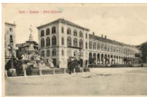
21707. * Split, Spalato; Hotel Bellevue, bank, foun 1400
