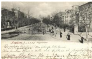
22313. ☒ Augsburg, Fuggerstrasse / street (EK) T21800
