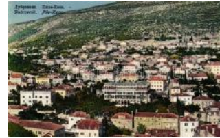
21666. ** Dubrovnik, Pile Kono T1/2 1200
