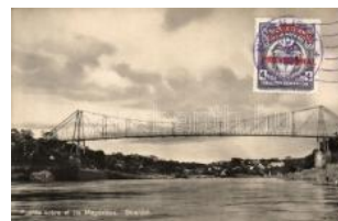
22893. * Girardot, bridge, Magdalena River T2 1000
