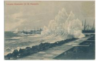
23361. * Colombo Breakwater (S.W. Mousson) T2 1200
