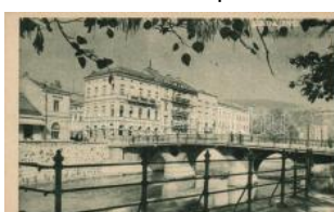
22579. ** Sarajevo, bridge T1/2 800
