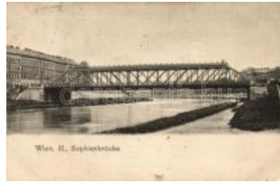
22531. Vienna, Wien III. Sophienbrücke / bridge (R 1800
