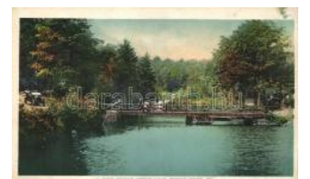
22453. ** Songo River, Maine, Sliding Bridge abov 900
