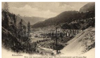
23029. ** Albula Railway, Landwasserviadukt, Switzerland 1000
