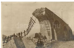
23563. ** Military WWI, destroyed bridge, photo 1400
