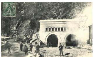
22822. ☒ Iselle tunnel (EK) T2/3 2400
