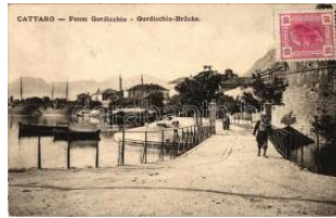
22608. ☒ Kotor, Cattaro, Ponte Gordicchio / bridge 1400
