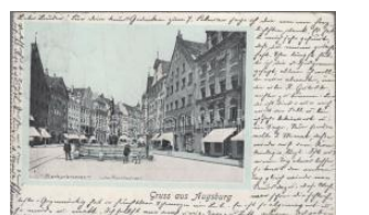
22649. ☒ Augsburg, Merkurbrunnen / fountain (EK) 1200
