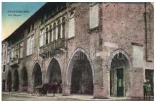
22887. ** Portogruaro, Via Cavour / street T2/3 1600
