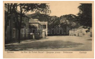
22605. ** Cetinje, Hofstrasse / royal palace street 2000
