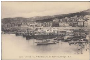
22138. ** Algiers, Alger; the commercial port, bou 1200
