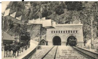
22940. ✱ Simplon Tunnel, horse cart, locomotive (R 5000
