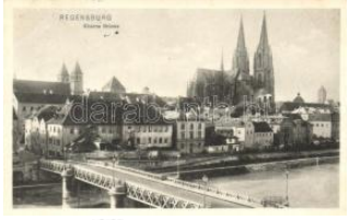
22754. ☒ Regensburg, Eisenbrücke / bridge T2 1400
