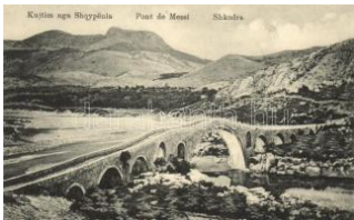
22130. ✱✱ Shkoder, Shkodra; Pont de Mess / bridge 2000
