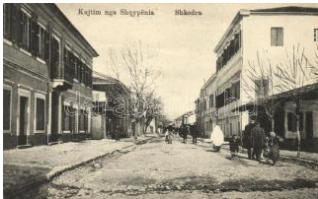
22127. ✱✱ Shkoder, Shkodra; street T1/2 2400
