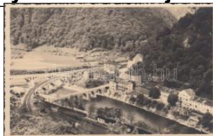
23132. * Zidani Most, bridge T1/2 1400
