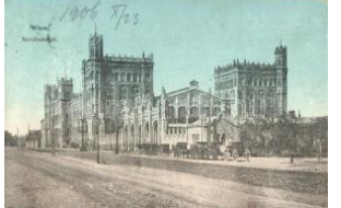
22173. ☒ Vienna, Wien II. N ordbahnhof / railway sta 1600
