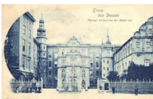
22613. ** Dessau castle (wet damage) T3/4 1400
