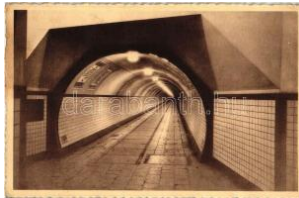
22221. ** Antwerpen, Anvers; Pedestrian tunnel u 1200
