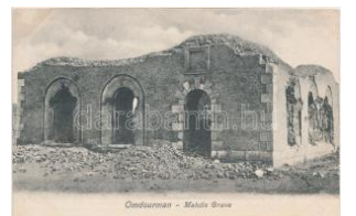
22877. Omdurman, Mahdis Grave (wet damage) 1200
