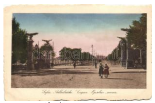
22264. ** Sofia, Adlerbrücke / bridge T2 1200
