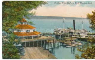
22060. Tacoma, Washington; pavilion, Point D 1200
