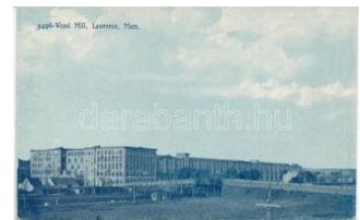
22231. ** Lawrence, Massachusetts; Wood Mill T1600
