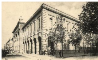
22878. ** Tunis, Hotel de Postes / Post office T1 1400
