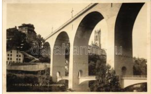
22818. ** Fribourg, Zaehringen bridge T1/2 1200
