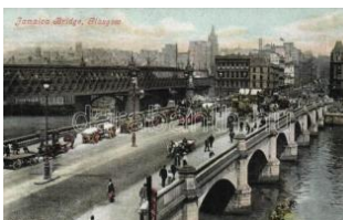
22600. ** Glasgow Jamaica bridge T1 1400
