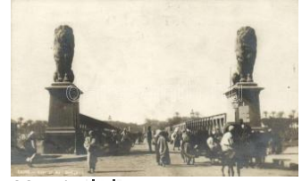
22471. *** Cairo, Kasr-El Nil bridge T2 1400
