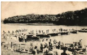
23464. K.u.K. Pioneer Battalion / temporary bridge 2000
