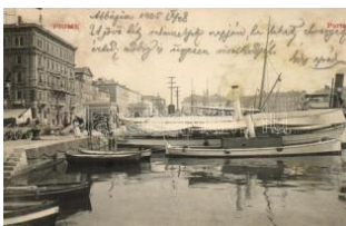
22024. ☒ Fiume, port, steamship (wet damage) T4 1000
