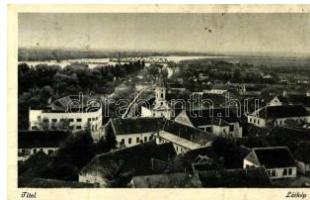
22118. ✳ Tittel, templom, híd / church, bridge T2 1200
