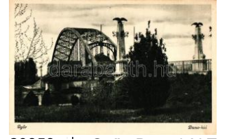
20858. ✳ Győr, Duna híd T1/2 1000
