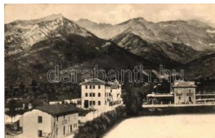
22808. ☒ Bardonecchia, Villa Ramazotti, Chalet G 2000
