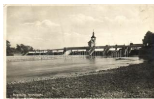
22277. ☒ Augsburg, Hochablass / water plant T2 1400
