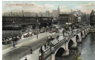
22262. ✳✳ Glasgow Jamaica bridge T1 1400
