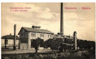
22564. * Mykolaiv, Nikolae v; Electric plant station 3800
