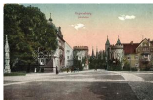
22370. ✱✱ Regensburg, Jakobstor / gate T2 1200
