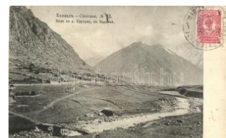
22439. ☒ Hurzuk river, Ka rachay district (fa) T3 1200
