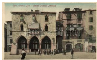
21814. * Split, Palazo Com unale / town hall, shop 1400
