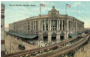
21917. ✱✱ Boston, Massachusetts; South Station ( 1400
