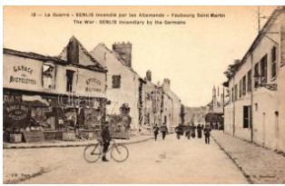
22019. ** Senlis, St. Martin, destroyed buildings 2200
