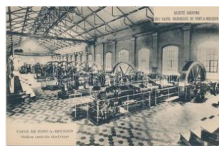
22013. ** Pont-a-Mousson, Station Centrale Elec 1800
