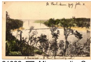
21932. ☒ Minneapolis, Gov ernment Dam, Locks (E 1400
