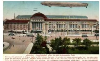
22610. Leipzig, Zeppelin, Hauptbahnhof / railway 1400
