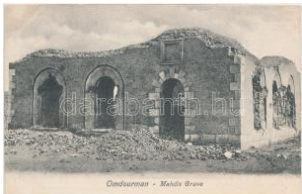
22799. ** Omdurman, Mahdis Grave (wet damag 1200
