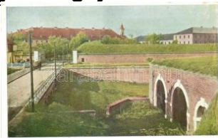
22220. ** Terezin, Bohusovicka brana / gates at 2600
