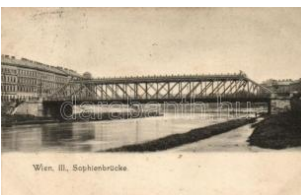
22107. * Vienna, Wien III. S. ophiëbrücke / bridge (R 1800
