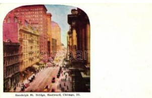
21895. ** Chicago, Rand olph St. Bridge T2 1200
