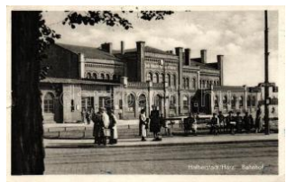
22335. ☒ Halberstadt, Bahnhof / railway station (b 1000
