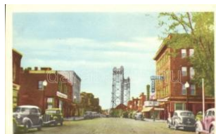
22271. * Welland, East Ma in Street and Lift Bridge 1200
