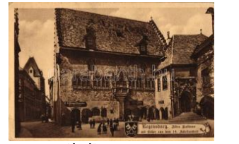
22779. ** Regensburg, Rathaus / town hall T2 1400
