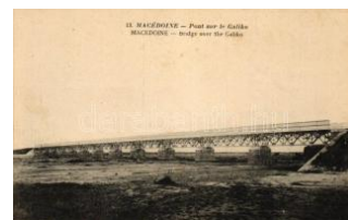
22535. * Macedonia, Bridge over the Galikos river 1600
