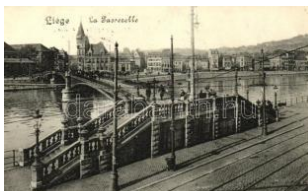
22306. Liege, Passerelle / bridge (EK) T2/3 1600
