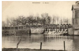
22453. Marconne, Le Moulin / mill, dam T1/2 2000
