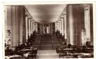
23358. ** Paquebot "Normandie" / interior, stairca 1400
