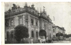
22159. ☒ Rzeszów, Sokol building T2 2200
