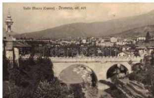
22432. ☒ Dronero, bridge (EK) T2/3 1200
