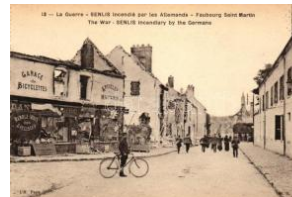
22053. Senlis, St. Martin, destroyed buildings 2200
