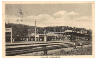
22341. ✳ Heringsdorf, Seeb ad / railway station (Rb) 2000
