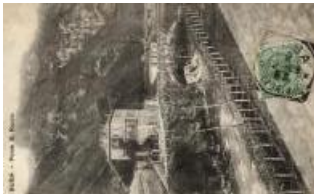
22494. ☒ Susa, Ponte S. Rocco / bridge T2 1200
