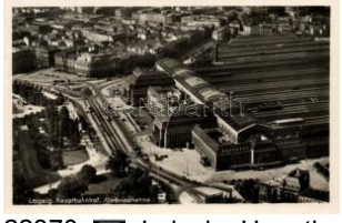
22370. Leipzig, Hauptbahnhof / railway station T 1400
