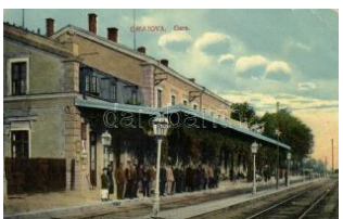
22550. Craiova, Gara / railway station (Rb) T3 5000
