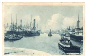
21720. ✳✳ Buenos Aires, D ique Tercero / third dam 1400
