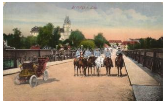
21893. ☒ Brandys nad Labem, bridge, soldiers on 3000
