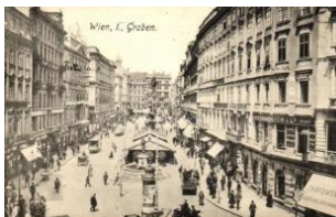
21857. * Vienna, Wien I. G raben, shop of Caldera 2000
