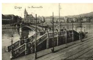
21897. ☒ Liège, Passerelle / bridge (EK) T2/3 1600
