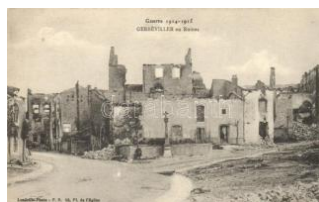
22026. ** Gerbéviller, destroyed buildings after th 2000
