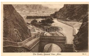
22304. ** Aden, Tanks T1/2 1400
