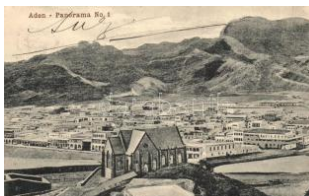
22309. ☒ Aden (wet damage) T4 900
