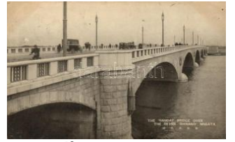
22263. * Niigata, Bandai Bridge over the Shinano 1800
