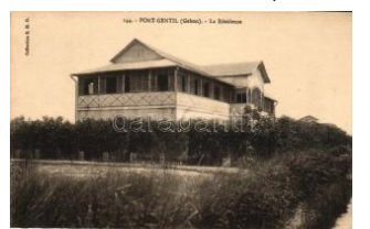
22123. ** Port-Gentil, residence T1 2600
