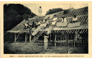
22124. ** Samkita, House construction T1 2400
