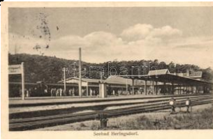
22330. * Heringsdorf, Seebad / railway station (Rb) 2000
