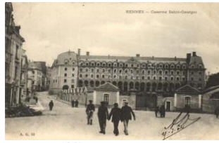
22122. Rennes, Caserne Saint-Georges / barrack 2200
