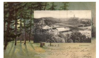
22323. Halle, Giebichentein / bridge, pine forest 3200
