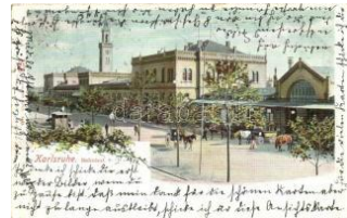
22335. ☒ Karlsruhe, Bahnhof / railway station (wet) 1900
