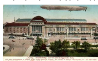
22355. ☒ Leipzig, Zeppelin, Hauptbahnhof / railway 1400
