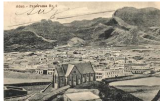
22321. ☒ Aden (wet damage) T4 900
