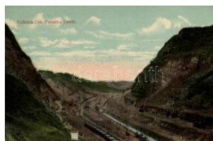
22789. ** Panama Canal, Culebra Cut T2 1600
