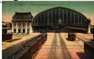
22092. ☒ Bordeaux, Gare d'Orléans / railway station, 3000
