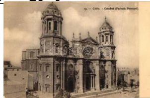
22797. ** Cádiz, Cathedra l, Main Facade (EK) T2 1400
