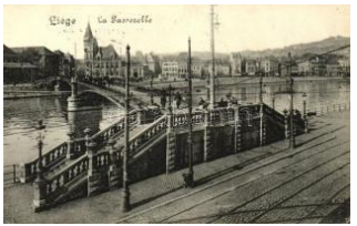
21971. 1 Liège, Passerelle / bridge (EK) T2/3 1600
