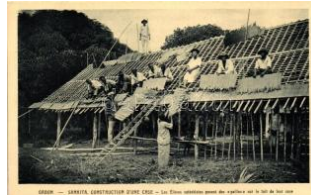
22161. ** Samkita, House construction T1 2400
