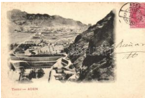
22377. Aden, Tanks (sm all tear) T3 1200
