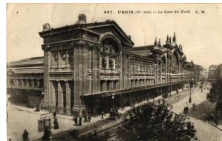
22280. ☒ Paris, La Gare du Nord / railway station ( 1400
