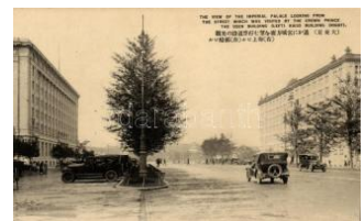
22350. ** Tokyo, Imperial palace, Kaijo building, 2200
