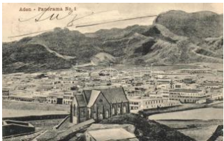
22375. Aden (wet damag e) T4 900
