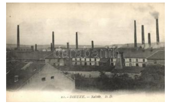
22252. * Dieuze, Saline / salt works, factory T2 3200
