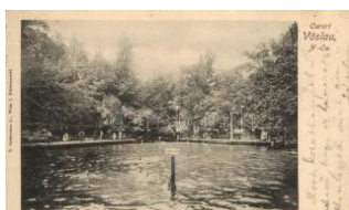
21896. ☒ Bad Vöslau, Bad / swimming pool (Rb) T 1400
