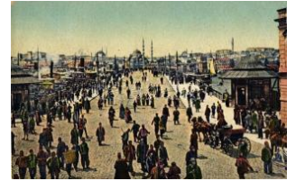
23129. ** Constantinople, New bridge T2 1200
