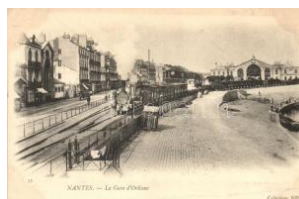
22288. ** Nantes, Orleans railway station, locom 2400
