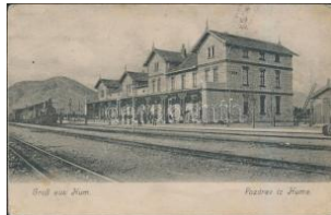
22087. Hum, railway station, locomotive (EB) T3 2200
