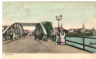
21874. Vinkovce, Vinkovci; bridge (wet damage 1000
