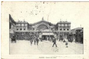
22322. ☒ Paris, 'Gare de l'Est' / Eastern railway sta 1800
