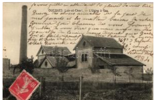
22304. ☒ Oucques, L'Usine a Gaz / Gas Factory T 5000
