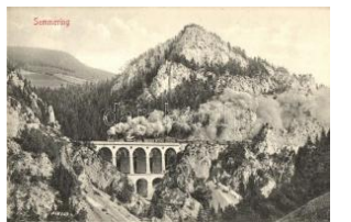
22026. ** Semmering, Via duct / railroad bridge T1 1000
