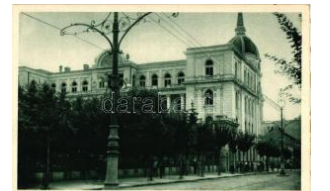
23105. ** Belgrade, Novi kralj dvor / courtyard (E) 1200
