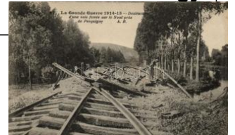
22357. * Picquigny, Pecquigny; Destruction of a railway 2400
