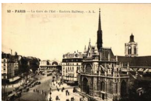
22342. ☒ Paris, Gare de l'Est / railway station T2 1400
