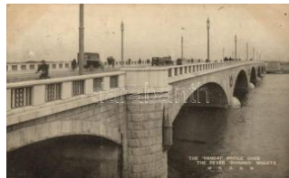
22523. * Niigata, Bandai Bridge over the Shinano 1800
