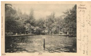
21787. ☒ Bad Vöslau, Bad / swimming pool (Rb) T2 1400
