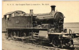
24282. G.W.R. Six Coupled Tank Locomotive No. 3000
