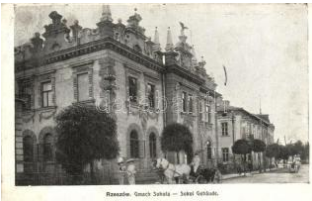
22240. ☒ Rzeszów, Sokol building T2 1000
