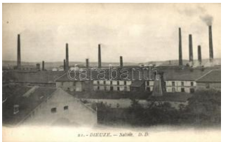
22148. ✨ Dieuze, Saline / salt works, factory T2 3200
