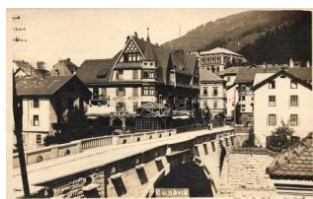
21840. * 1924 Landeck, Hotel Post, bridge, photo T 1200
