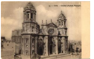
22664. ** Cadiz, Cathedral, Main Facade (EK) T2 1400
