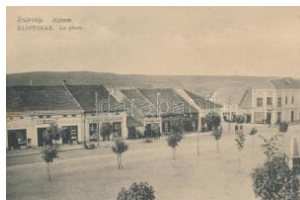
22895. ✱ Zajecar, Main square, monument, shop o 2400
