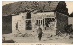
22228. ** Carnoy, destroyed houses after the bom 2000
