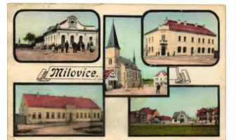
22204. Milovice; multi view, hotel, church (Rb) T 1000
