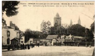
22362. Senlis, WWI destroyed buildings, Avenue 1800
