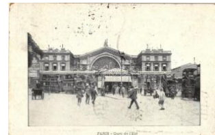
22300. Paris, 'Gare de l'Est' / Eastern railway sta 1800
