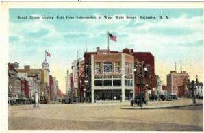
22093. ** Rochester, Br oad street looking east 1200
