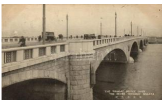
22465. * Niigata, Bandai Bridge over the Shinano 1800
