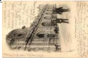
22287. Orleans, 'Nouvelle Gare' / new railway st 2000
