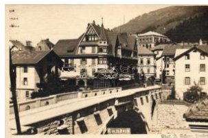
21555. 1924 Landeck, Hotel Post, bridge, photo T 1200
