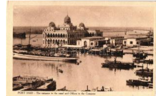
21756. ** Port Said, entra nce to the canal, offices 1000
