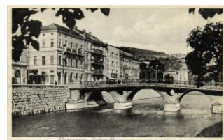
21672. Sarajevo, Princip Brücke / bridge (EK) 1200
