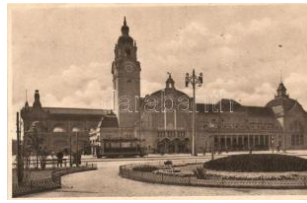
22399. ** Wiesbaden, Hauptbahnhof, railway stati 1200
