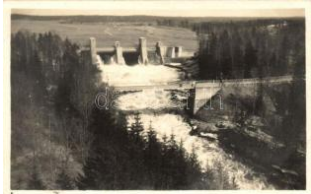
22009. ** Imatra, river dam, bridge T2 1400
