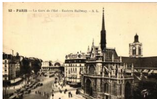
22101. ☒ Paris, Gare de l'Est / railway station T2 1400
