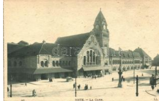
22066. ** Metz, La Gare / railway station, terminus 2000
