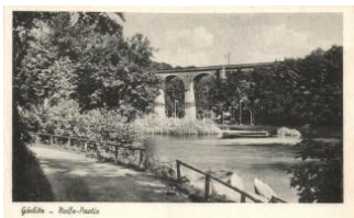
22297. ** Görlitz, Neisse-Partie / riverside, railwa 1200
