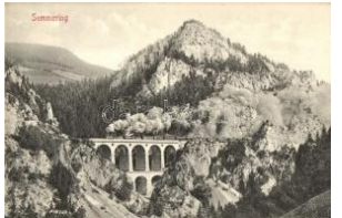
21907. ** Semmering, Viadukt / railroad bridge T1 1000
