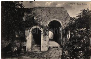
22537. ** Pompei, 'Porta Marina' / Seaside gate 1400
