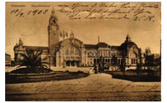
22400. ☒ Wiesbaden, Hauptbahnhof / main railway 1400
