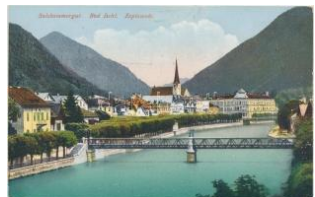
22313. ☒ Bad Ischl, Esplanade / bridge T2 1200
