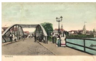
22215. ☒ Vinkovce, Vinkovci; bridge (wet damage) 1000
