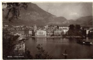
22864. 1 Riva del Garda, P anorama / general view 1200
