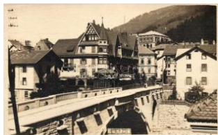
22345. * 1924 Landeck, Hotel Post, bridge, photo T1200
