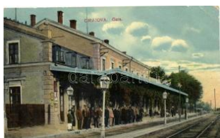
22933. * Craiova, Gara / railway station (Rb) T3 4000
