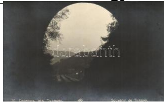
22456. ** Veliko Tarnovo, Tarnovo; railway tunnel 1400
