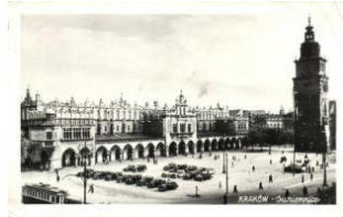
22621. * Kraków, Sukiennice / main square, Krakó 1400
