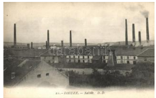
21693. * Dieuze, Saline, salt works, factory T2 3200
