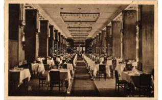
21878. ** Berlin, Weinhaus "Rheingold", Pfeiler S 1600
