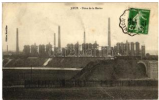
21707. ☒ Joazeuf, Usine de la Marine / marine factory 5000
