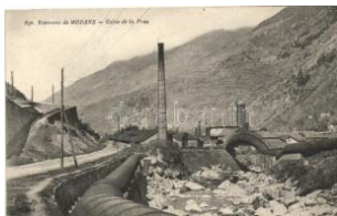
21733. ** Modane, Usine de la Praz / factory T2 2000
