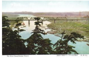
21821. ** Tokyo, Tama river, bridge T2 1400
