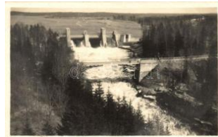
21662. ** Imatra, river dam, bridge T2 1400
