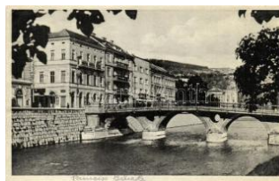
21750. Sarajevo, Princip Brücke / bridge (EK) 1200
