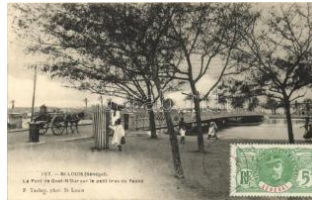
22638. * Saint-Louis, Pont de Guet-N'Dar / bridge 1400
