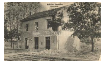
21884. ✳✳ Dontrien; railway station damaged duri 1600
