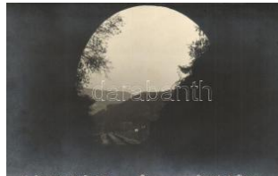
21767. *** Veliko Tarnovo, Tarnovo; railway tunnel 1400
