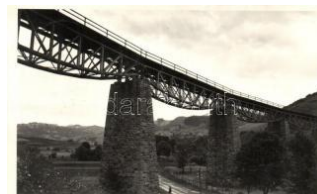
21384. ☒ Uzsok, Uzhok; Viadukt / viaduct, 'Sport Sz 800
