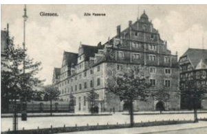
22233. ** Giessen, Alte Kaserne / old barracks, G1800
