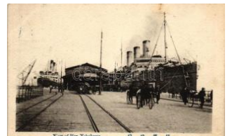
22024. * Yokohama, Pier T2 1600
