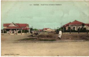
22629. ** Dakar, Rond Point at Avenue Gambetta 1400
