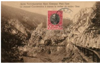
21853. Cestobrodica, river, tunnel (EK) T2/3 1200
