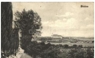
21301. Stainz, general view (EK) T2/3 1000
