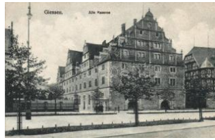
21618. ** Giessen, Alte Kaserne / old barracks, G1800
