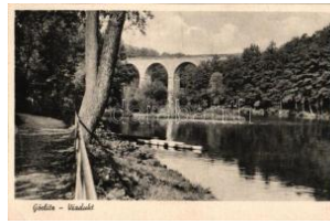
21619. ** Görlitz, railway viaduct between Germa 1400
