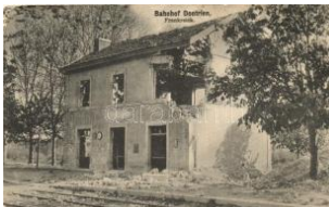
21429. ** Dontrien; railwa y station damaged duri 1600
