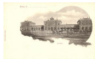
21724. ✱✱ Reims, La Gare / railway station, horse 3000
