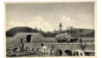
21608. * Terezín, tunnel T2 / 3 1200
