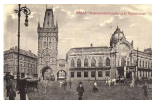
21595. * Praha, Prag; Reparaentationshaus b. P 2000
