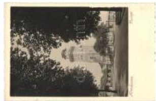
21931. * Frohnau, Turm / clock tower T2 1200
