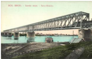
21537. ** Bosanski Brod, Savski most / bridge, lo2000
