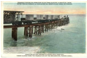
22373. * Panama Canal, Droppong 25 ton concret 1600
