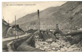
21662. ** Modane, Usine de la Praz / factory T2 2000
