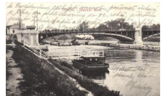
21600. ☒ Praha, Prag; Hlávka most / bridge T2 1400
