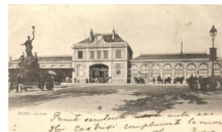
21778. ☒ Vichy, La Gare / railway station (EK) T2/ 3000
