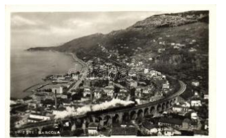
22266. ** Trieste, Barcola; railway viaduct with lo 1600
