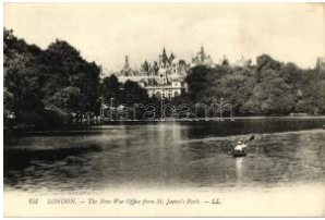
21895. ** London, The New War Office from St. James's Park 1200
