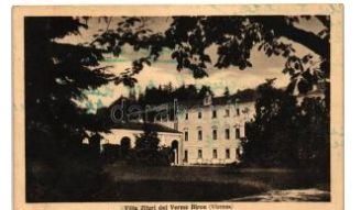
22062. Biron, Villa Zileri (wet damage) T3/4 1400
