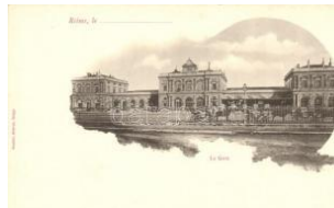
21764. ** Reims, La Gare / railway station, horse 3000
