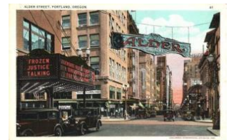
21486. ** Portland, Orego n. Alder Street, Alder The 800
