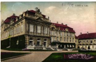
21579. ✨ Lysá nad Labem (wet damage) T4 1000
