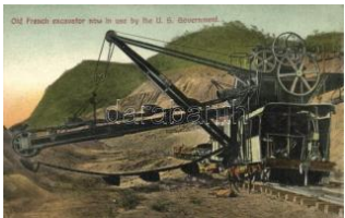
21959. * Panama, old French excavator now in us 3000
