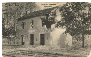
21616. ** Dontrien; railway station damaged duri 1600
