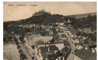
20994. ☒ Kőhalom, Reps; (ázott / wet damage) T4 1600
