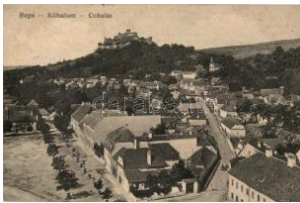
20980. ☒ Köhalom, Reps; (á zott / wet damage) T4 1600
