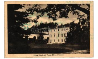
21705. Biron, Villa Zileri (wet damage) T3/4 1400
