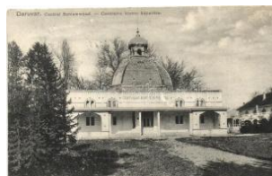
21239. * Daruvár, Daruvar; Central Schlambad, 1400
