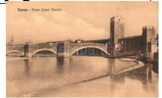
21857. ** Verona, Ponte Castel Vecchio / bridge T 1400
