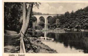
21827. ** Görlitz, railway viaduct between Germa 1400
