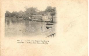
21737. Erode, Cauvery Bridge (EB) T3/4 1600
