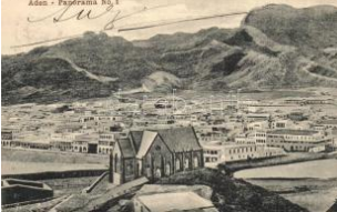
21753. Aden (wet damag e) T4 900
