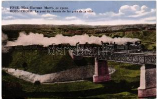
21575. ** Ruse, Roustchouk; railway bridge, loco 3000
