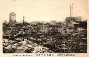
21771. ** Tokyo, The Great at Kanto earthquake; K 2600
