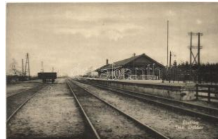
21741. * * Den Dolder, railway station (fl) T2/3 1000
