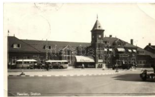
21744. * 1947 Heerlen, Station / railway station (E 1400
