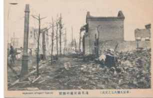
21772. ** Tokyo, The Great at Kanto earthquake; K 2600
