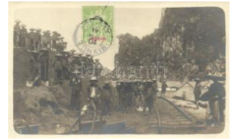
22062. ✳ Tonkin region, Ra ilroad construction, pho 5500
