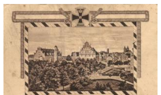
22020. Wittenberg (wet damage) T4 1000
