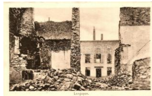
21774. Longuyon, bombed building, ruins T 1200
