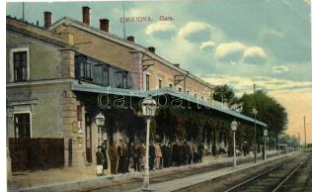
22162. * Craiova, Gara / railway station (Rb) T3 2200
