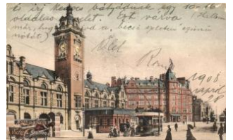
21908. ☒ Nottingham, Victoria Station, tram (EK) T 2000
