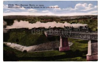
21552. ** Ruse, Roustchouk; railway bridge, loco 3000
