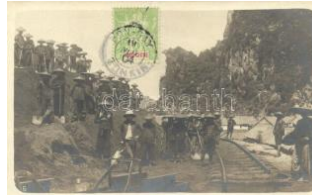
22027. * Tonkin region, Railroad construction, photo 5500
