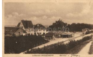
21899. * Wassenberg, Bahnhof / railway station (E) 2800
