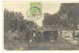
21492. * Tonkin region, Ra ilroad construction, pho 5500
