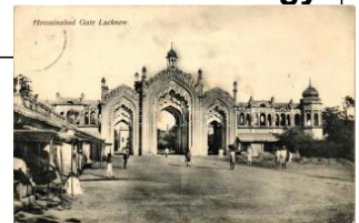
21221. Lucknow, Hossainabad Gate T2 2000
