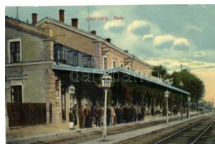
21444. ✳ Craiova, Gara / railway station (Rb) T3 2000
