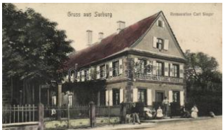
21198. ☒ Surbourg, Surbur g; Restauration Carl Sin4600
