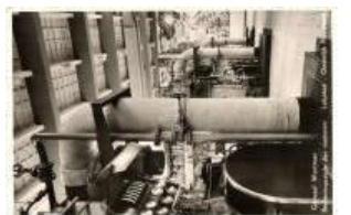
21823. ☒ Lelystad, Gemaa l Wortman / pumping st 1000
