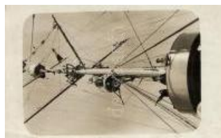
22386. ** Sailors of the mast, photo (EK) T2/3 1600
