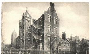
21912. Kensington, The Infirmary, hospital (fro 2000 )
