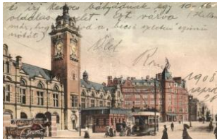
21926. ☒ Nottingham, Victoria Station, tram (EK) T — 2000
