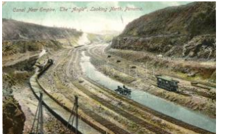
22020. * Panama, Canal near Empire, The Angle 1800
