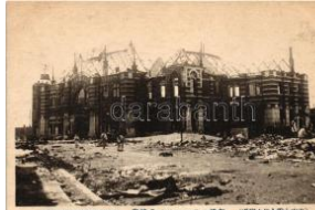
21758. ** Tokyo, The Gre at Kanto earthquake; S 2600
