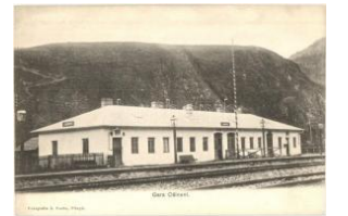
22035. Caineni, Gara C aineni / railway station 7000
