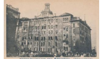
21755. ** Tokyo, The Gre at Kanto earthquake; M 2600
