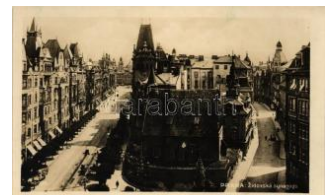
21635. ** Praha, Zidovska synagoga / synagogue 3000
