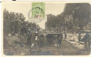
22125. * Tonkin region, Ra ilroad construction, pho 5500
