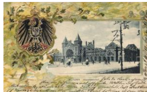
21881. ☒ Altona, Hauptbahnhof / railway station, c 3000
