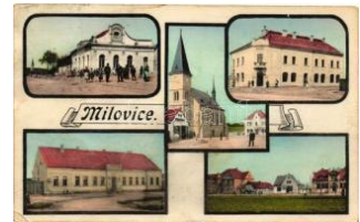
21810. * Milovice; multi view, hotel, church (Rb) T 1000
