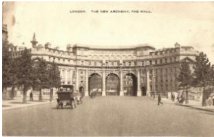
22260. ☒ London, The New Archway, the Mall T2/3 1000
