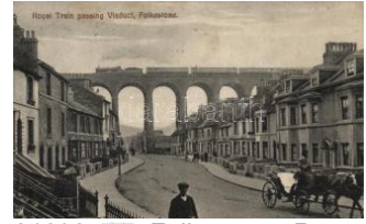
21690. ☒ Folkestone, Royal Train passing Viaduct 1200
