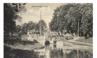
21746. ** Borensbergs Sluss, SS "Per Brahe" stea 800
