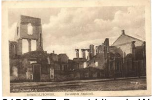
21583. Brest-Litovsk, Wa r damaged buildings T2 2600
