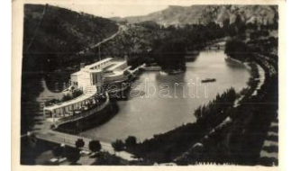
21758. * Ankara, Angora; Baraj / dam, photo (EK) 1000
